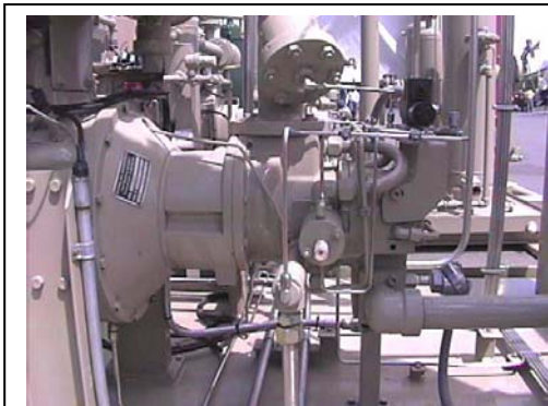
Figure 14- HG12 showing one of two Versatrol pockets. Second identical pocket is on the opposite side
